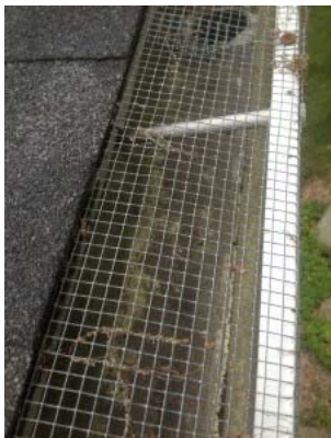
Gutter screen installed left. Tin snips, screws, pry bar center. Truss head screws \frac{1}{2} " right.
